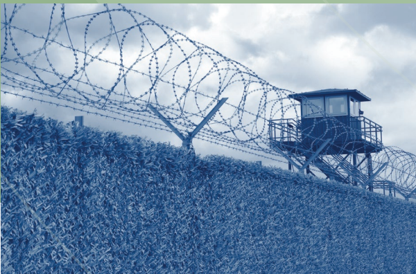
A single ReGuard radar is capable of covering up to 22 km of the border.
